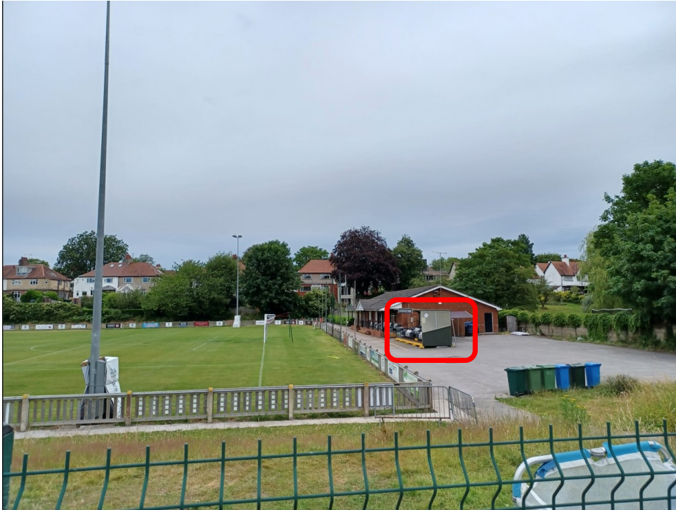
View northwards from external path to the south of site, stand is edged in red
